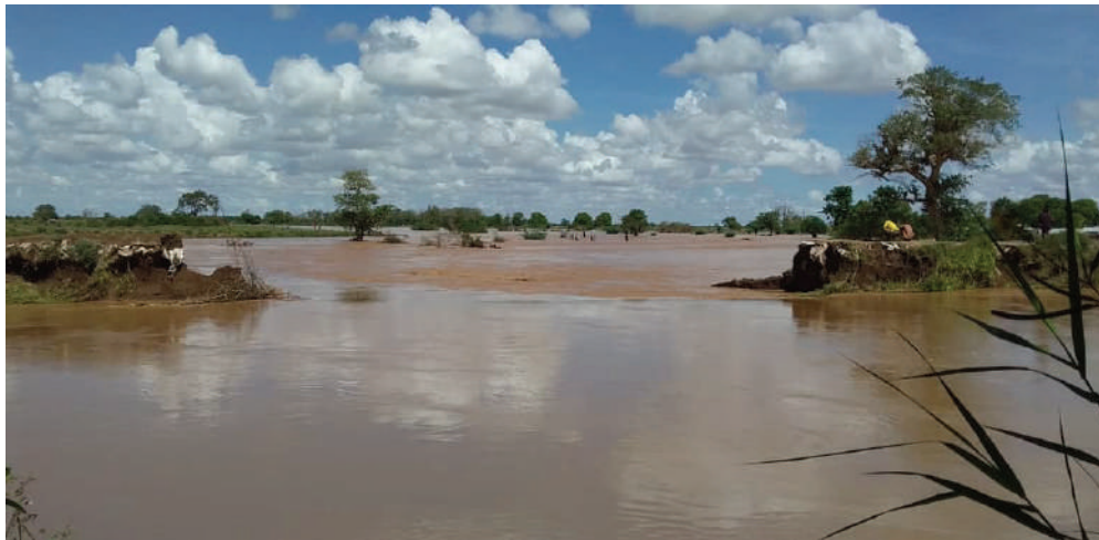
Figure 5.11: Deliberate embankment breach for irrigation purposes
