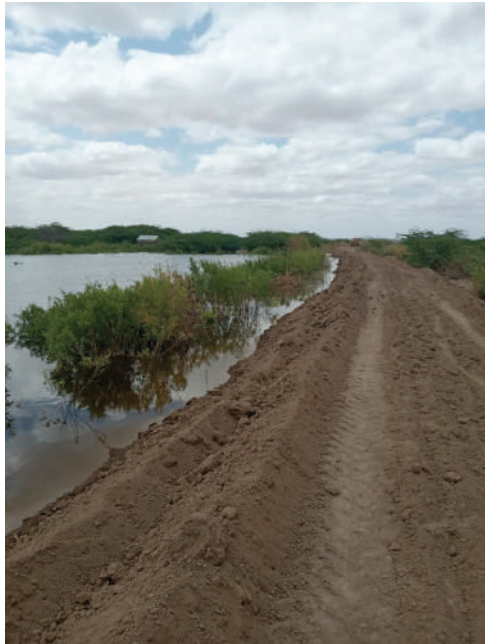
Figure 5.4: Dike (in combination with a road) constructed perpendicular to the Shabelle upstream of Beledweyne
