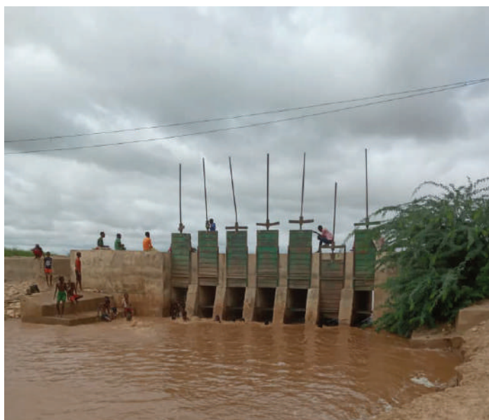
Figure 5.7: Intake structure for the flood by-pass in Beledweyne requiring maintenance, before the partial rehabilitation in 2020
