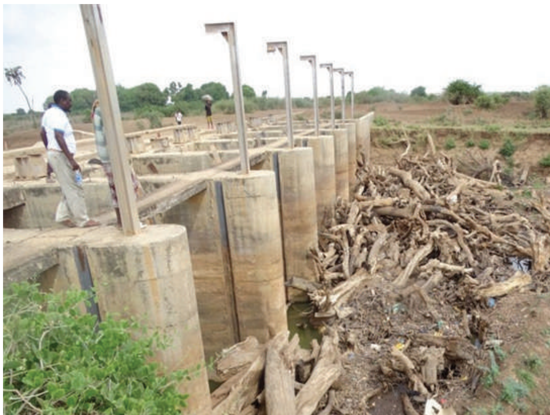
Figure 5.14: Sabuun barrage; without steel gates, water levels are controlled by wooden debris
