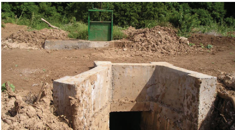
Figure 5.12: Small irrigation channel equipped with a gate
